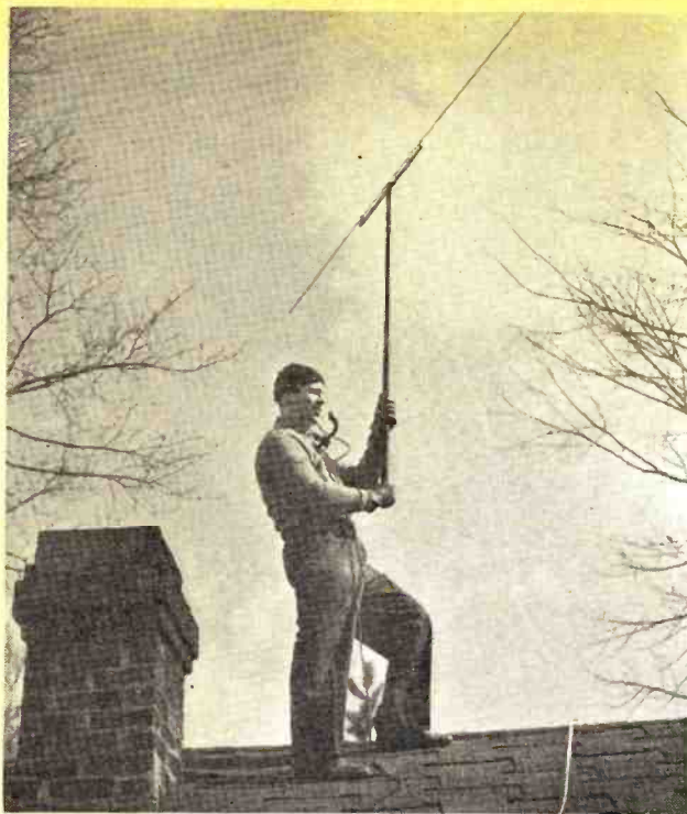
Fig. 1. The best location for television antenna is determined by testing various roof positions with a portable probing dipole, connected to the television set. Results are communicated to technician on roof by means of a telephone network.
